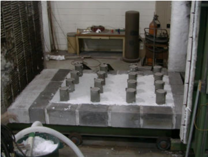
After the Foamfrax Insulation was gunned into place, a wet trowel was used to work the material around the support piers and smooth the surface of the car deck. The result was a monolithic, energy efficient insulation system, which was installed very fast. This allowed the customer to return the furnace to service quickly.
