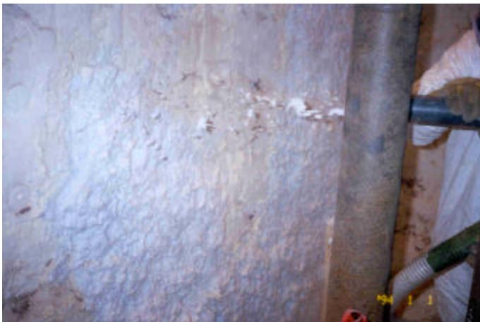
For optimal adhesion, the ceramic fiber substrate must be pre-wet with water before the Foamfrax is applied. In this instance, the anchoring hardware for the layered blanket lining was left in place and actually helps secure the Foamfrax Insulation.
