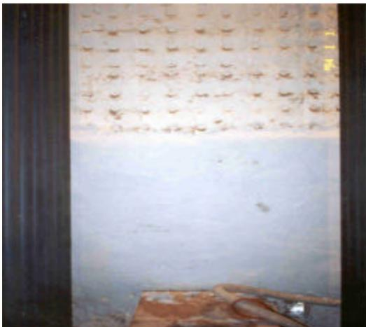
On vertical surfaces over existing refractory, troweling of the Foamfrax Insulation surface is optional. In this instance, a light layer of low density (very foamy) Foamfrax Insulation was applied and troweled smooth to finish the surface.
