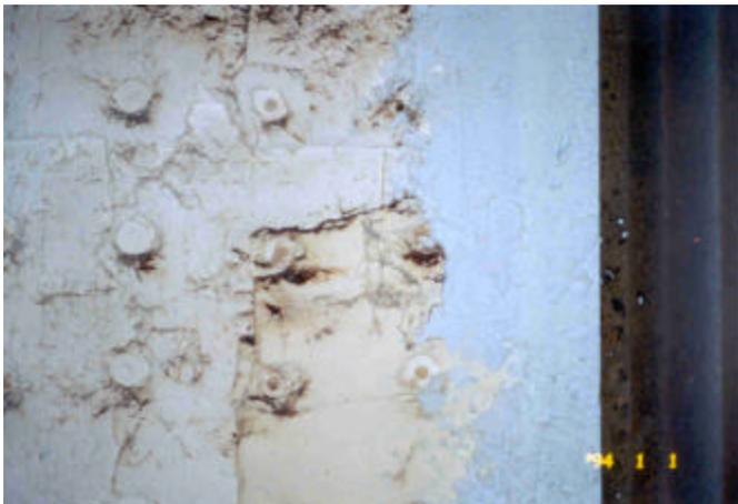
After years of service, the hot face lining of this ammonia reformer had become devitrified and loose in some areas. Prior to the application of the Foamfrax Insulation, all loose/hanging fiber was removed. For the removal of any after service refractory material, refer to the product MSDS for proper material handling guidelines.
