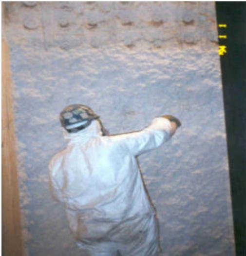
The installation of Foamfrax Insulation allowed the customer to immediately put the reformer back on line. It was also a more economical option to removing and replacing the entire hot face layer of blanket and afforded the customer increased insulating value with the additional 3” of Foamfrax Insulation.
