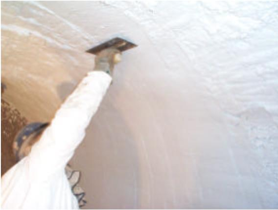
After the Foamfrax lining veneer has been installed, use a trowel to smooth the finished surface. Occasionally wetting the trowel allows it to flow freely over the Foamfrax material as it is troweled. Note: There is no critical heat-up/cure-out for Foamfrax Insulation. This unit was put into service immediately after installation, using the customer's normal start up procedure.
